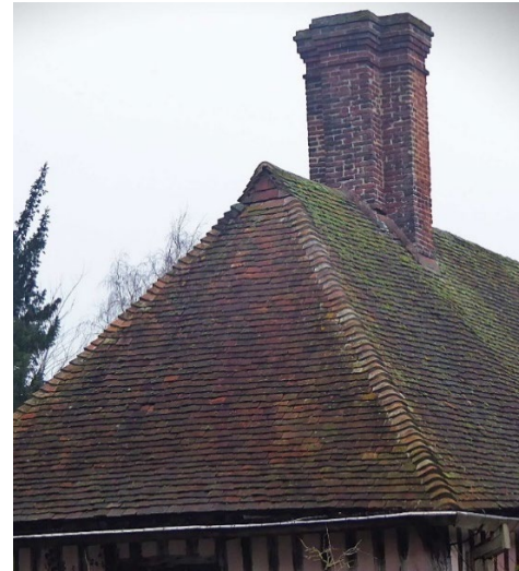
Figure 28: Clay roof tiles
