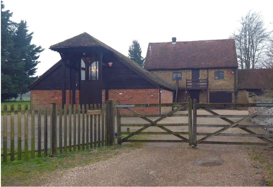
Figure 11: The glass workshop in the foreground and the agricultural building behind
