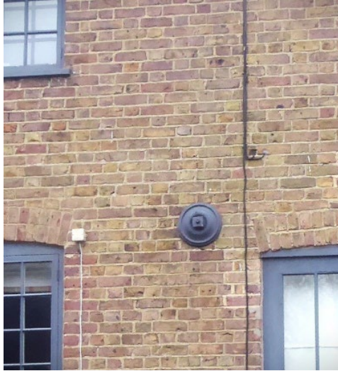
Figure 23: Nineteenth-century stock bricks at Bexon Manor Oast House
