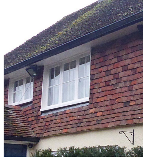
Figure 24: Hanging tiles on Yew Tree Cottage
