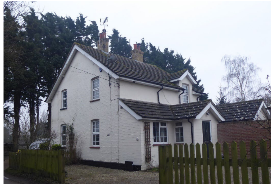
Figure 18: Bexon Manor Cottages
