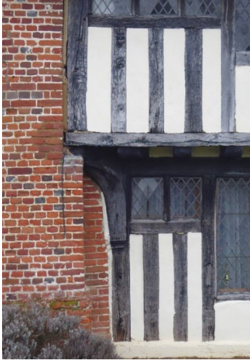
Figure 22: Close studding and a jettied first floor at Bexon Court
